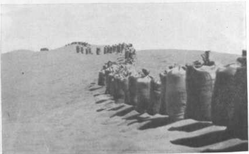
FIGURE 5.—Gunny sacks placed on the crest of dunes act as wind deflectors and lower as the wind removes the sand from under them.
